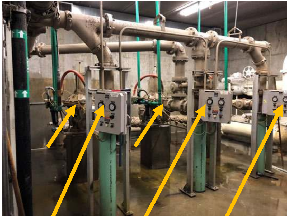
Electrical Panel Replacements (pre-installation)
