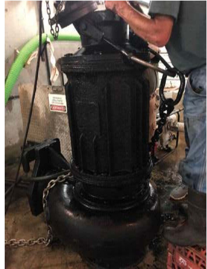
Submersible pump upon inspection
