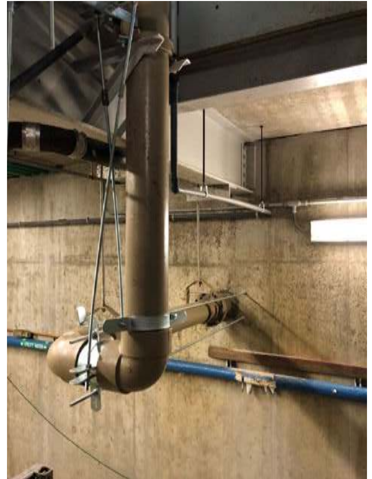
Reinforcement Rods Installed Post-Event
