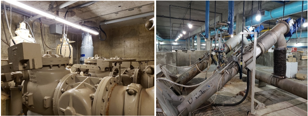
Figure 1. Left: Two Fairbanks Morse (Tan), New Flygt (Gray) Pumps. Right: Rotary Screens.
