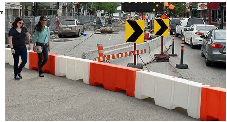
Pedestrian Channelizer using a Temporary Barrier
