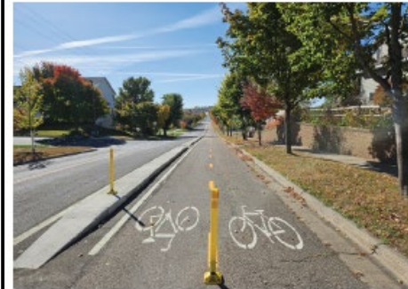
On-street cycle track along Maple St
